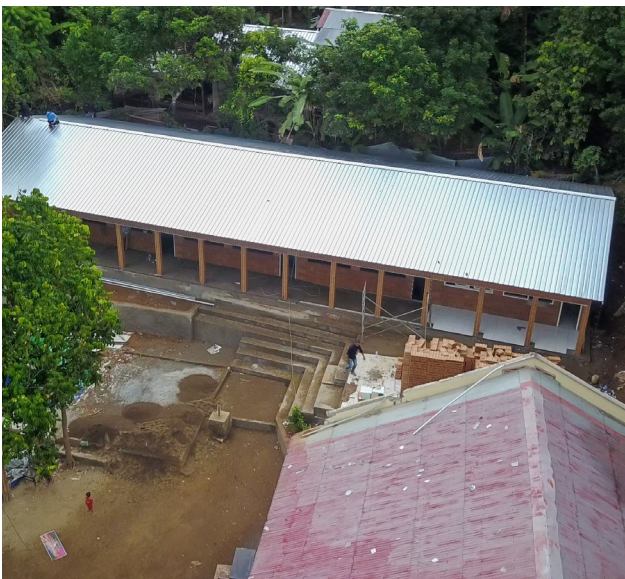
Figure 3: The first Block School constructed in Taman Sari, Lombok
